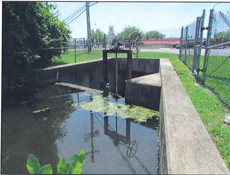
Photo 25 (06/24/14): Bypass Canal Spillway Leading to Underground Canal
