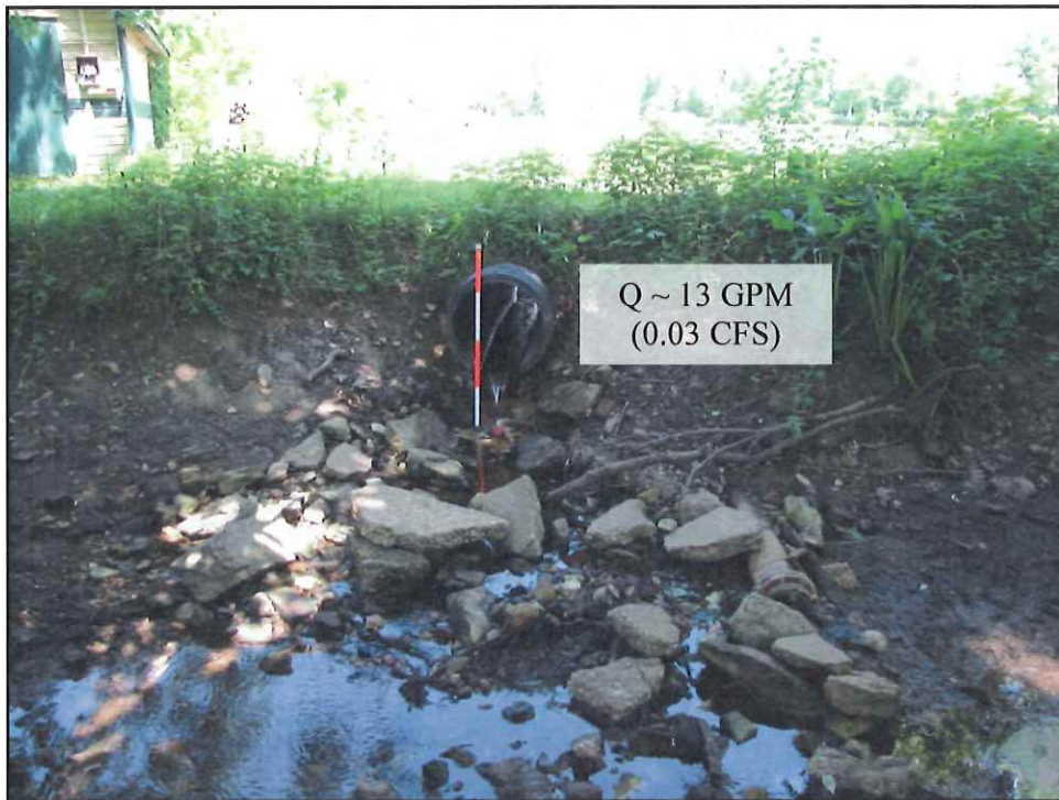
Photo 23 (05/31/13): Downstream HDPE Pipe from Lake 1 to Bypass Canal
