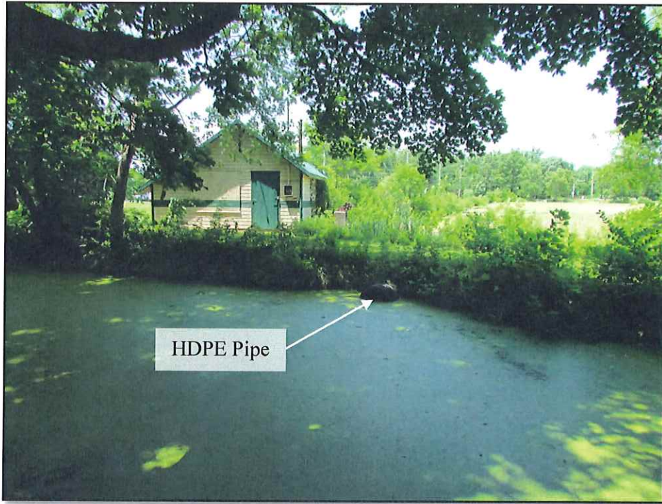
Photo 24 (06/24/14): Downstream HDPE Pipe from Lake 1 to Bypass Canal
