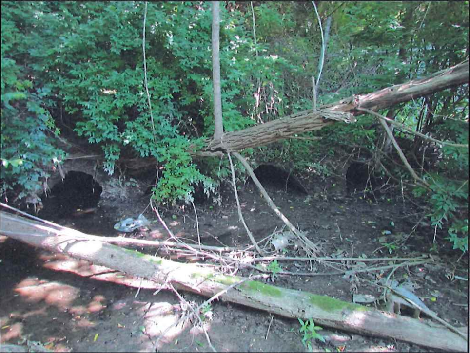
Photo 13 (06/24/14): Corrugated Metal Pipe Culverts Beneath Route 30
