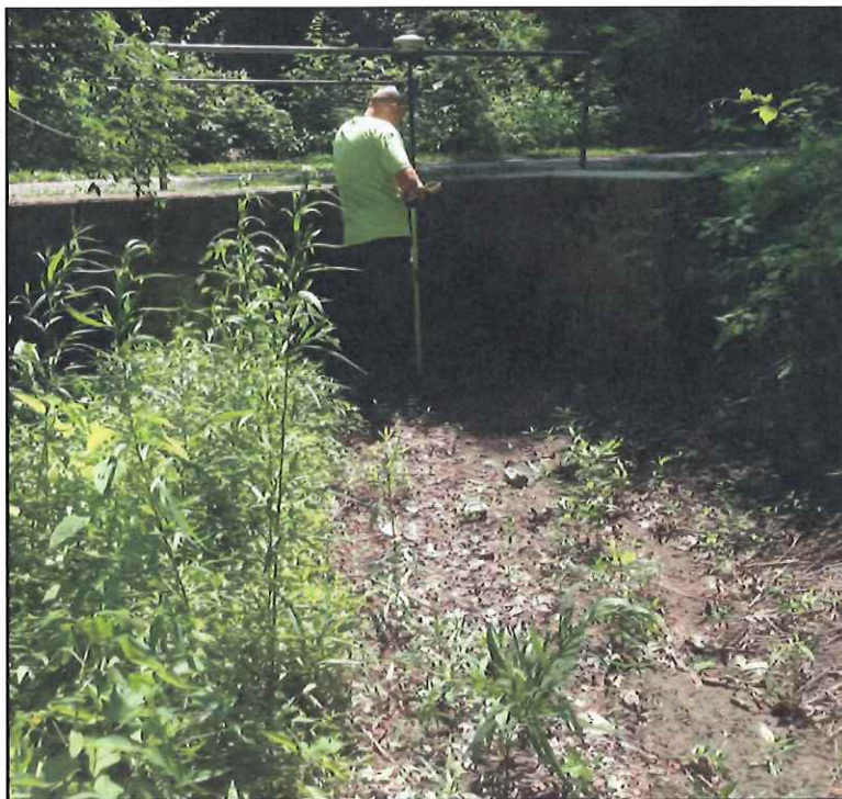
Photo 11 (06/24/14): Struble Trail Crossing Over Canal (North of Route 30)
