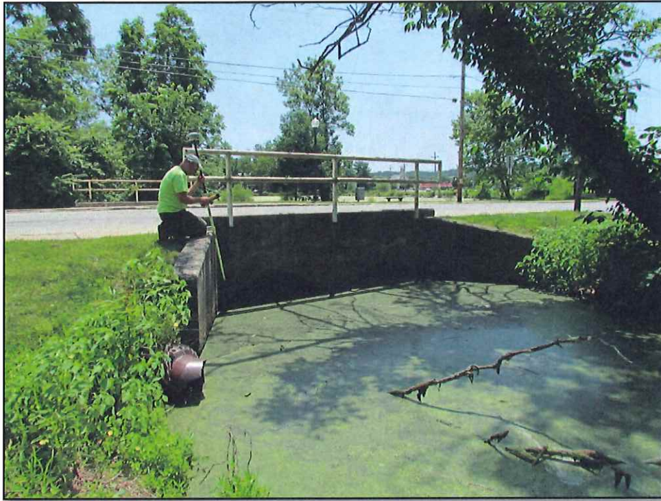
Photo 20 (06/24/14): Culverts Beneath E. Pennsylvania Ave.
