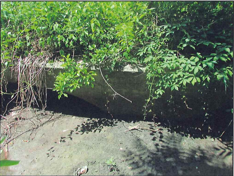
Photo 17 (06/24/14): Discharge End of Concrete Culverts Beneath Norwood Rd.
