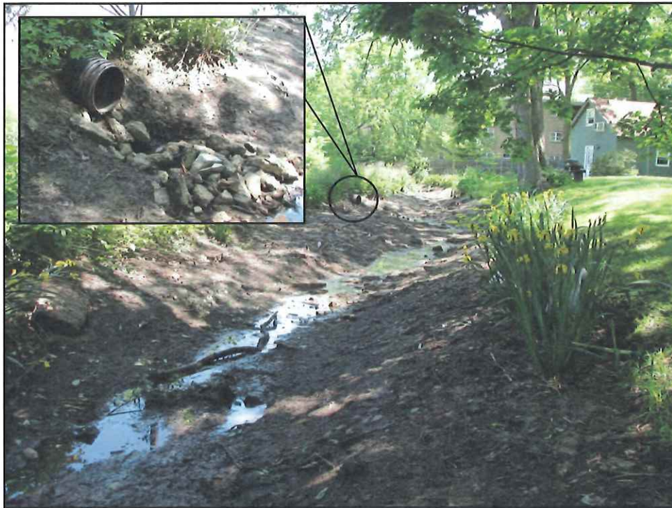
Photo 22 (05/31/13): Upstream HDPE Pipe from Lake 1 to Bypass Canal
