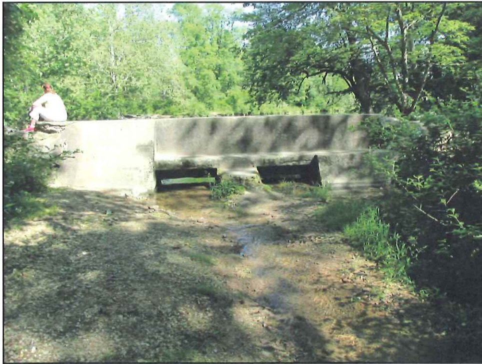
Photo 3 (05/31/13): Downstream End of Canal Intake (Looking Upstream)
