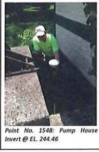
Point No. 1548: Pump House Invert @ EL. 244.46
