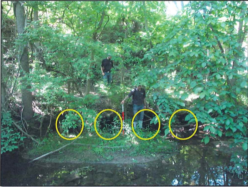
Photo 12 (05/31/13): Corrugated Metal Pipe Culverts Beneath Route 30
