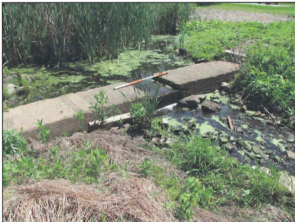
Photo 19 (05/31/13): Weir Discharge at Lake 2
