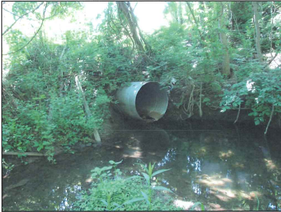
Photo 14 (05/31/13): Example of Stormwater Discharge into Canal
