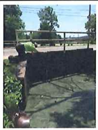
Point No. 1547: Invert of pipe @ EL. 244.60
