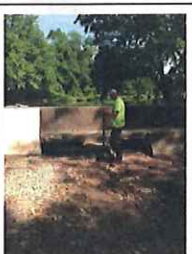
Point No. 1536: Invert @ Canal Entrance @ EL. 250.22
