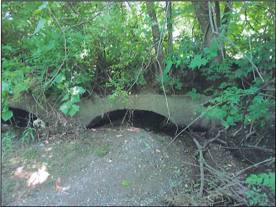
Photo 16 (06/24/14): Intake Side of Concrete Culverts Beneath Norwood Rd.
