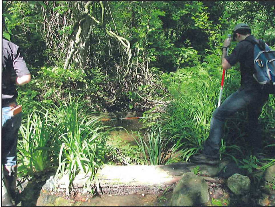
Photo 8 (05/31/14): Concrete Sill ~170-FT Downstream of Canal Intake
