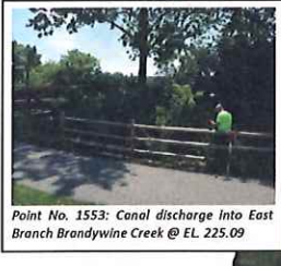
Point No. 1553: Canal discharge into East Branch Brandywine Creek @ EL. 225.09
