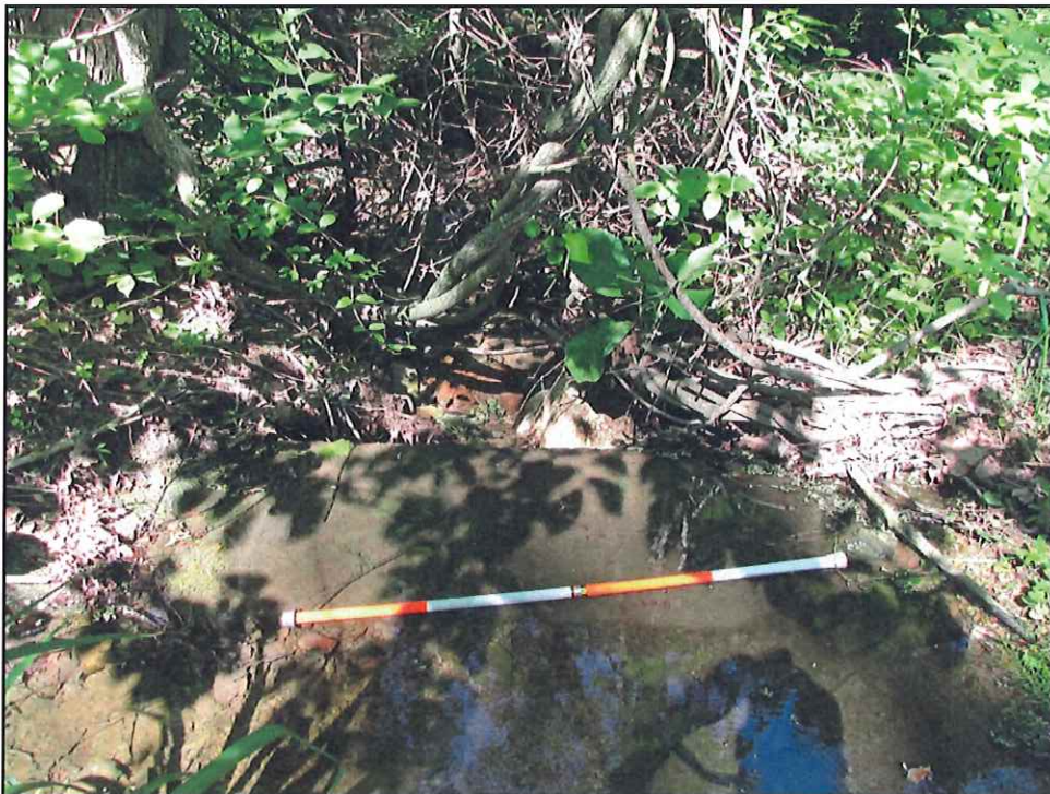
Photo 9 (05/31/13): Close-up of Concrete Sill
