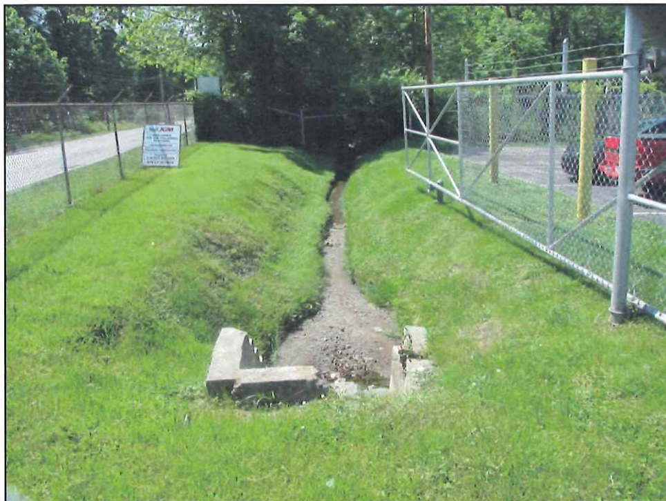
Photo 15 (05/31/13): Example of Stormwater Discharge into Canal
