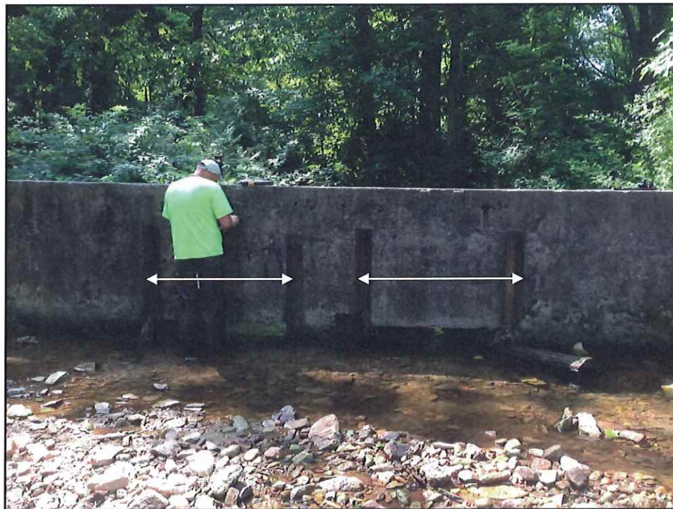
Photo 2 (06/24/14): Two Intakes into Canal
