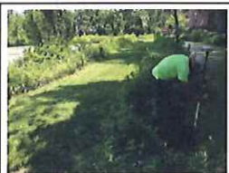
Point No. 1550: HDPE Invert @ EL. 245.86
