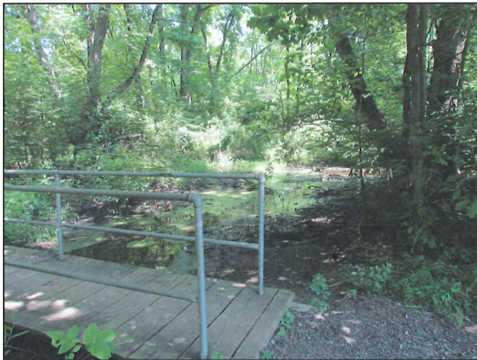
Photo 18 (06/24/14): Footbridge Over Canal Between Lake 4 and Lake 3
